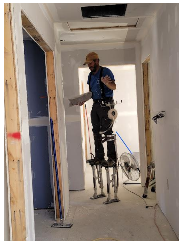
Tim mudding the walls
